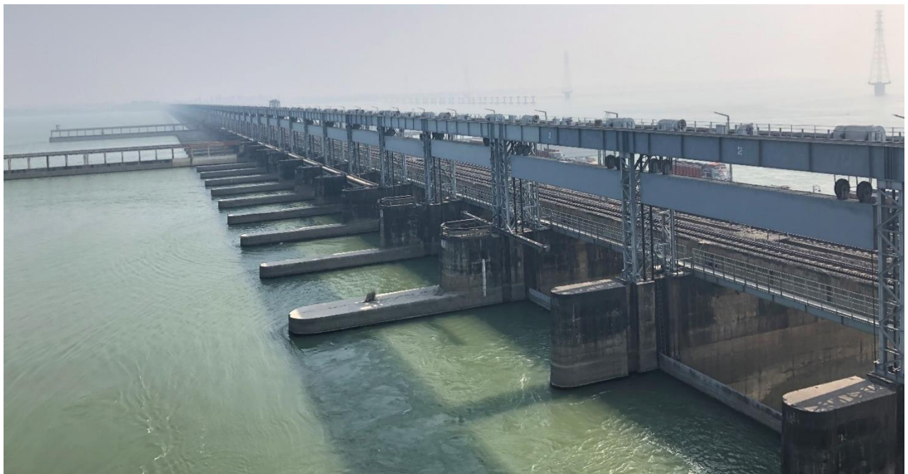
Fig. 5.10: Farakka Barrage Project- Main Barrage- Upstream view
