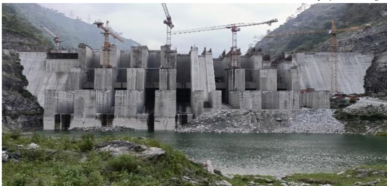
Fig. 5.4: Punatsangchhu-II Concrete Gravity Dam
