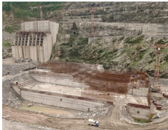
Fig. 5.3: Dam Construction site of Arun-3 HEP
