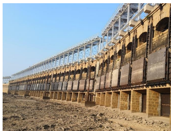
Fig. 5.7: Krishna Raja Sagara Dam- Upstream view- Gates at two level
