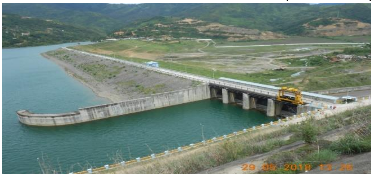
Fig. 2.4: Thoubal Multipurpose Project, Manipur (Project under PMKSY-AIBP)
