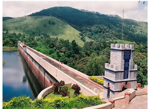
Fig. 5.14: Mulla Periyar Dam
