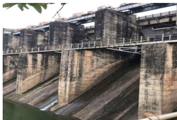
Fig. 5.13: Spillway of Sondur Dam
