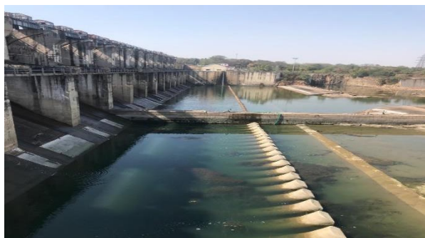
Fig. 5.12: Energy Dissipation Arrangement of Ravisankar Sagar Dam
