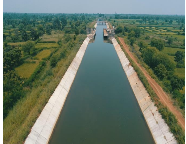
Fig. 8.2: Gosikhurd (National) Project, Maharashtra (under PMKSY-AIBP)
